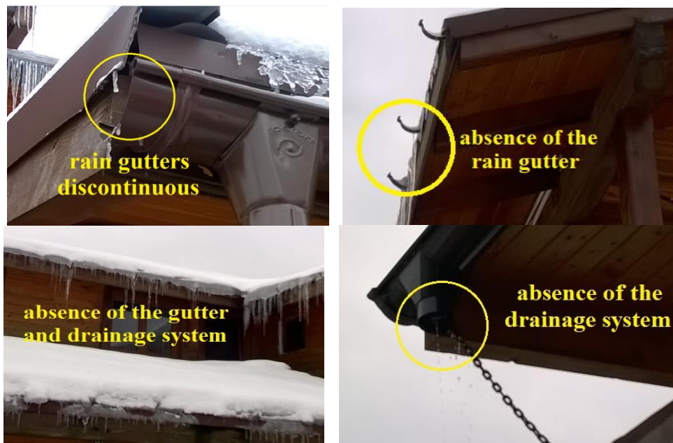
Fig. 2. Highlights of the technical state of the meteorological water collection and evacuation system
